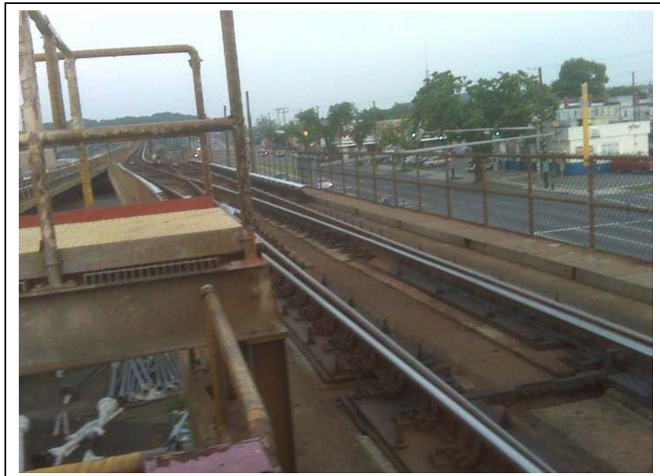
Picture 4 - D & G Platform, Track 1
