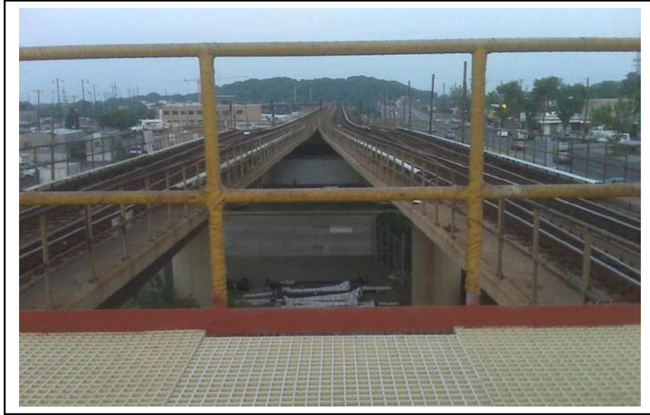
Picture 3 - D & G Platform facing Benning Road portal and Minnesota Avenue aerial structure.
